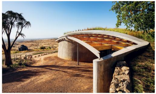
cast and shaped around pre-existing site features using flexible formwork. A granite aggregate from a local quarry was added to the concrete mix and the surface was ground down to a finely textured finish that delicately exposes the aggregate. Sections of the floor emulate the rich red sand of the Kalahari.
